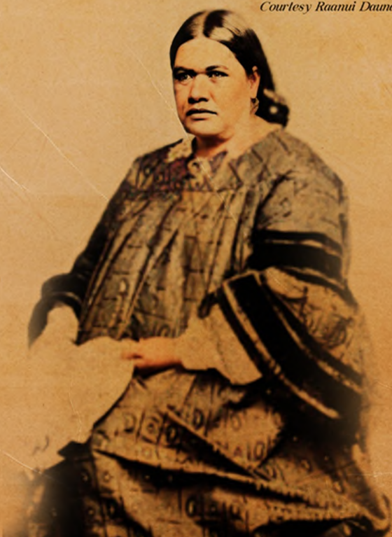
Ari'itaimai Courtesy Raamui Damassans
